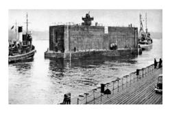
operation to maintain a never-ending supply of everything required to carry the war onto Berlin. This included the formation of the Mulberry Harbours which were massive temporary landing stages erected to supply the allied armies. This photo shows a section of Mulberry being towed by tugboats.
